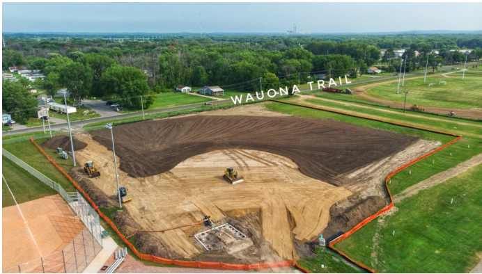
Drone picture of new ball field construction (Courtesy of Joshua Banks)
